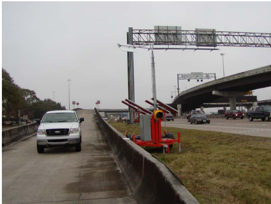
Figure 7. Mobile AVI Violation Enforcement Unit US-290 HOV Lane – Dacoma Exit Ramp
