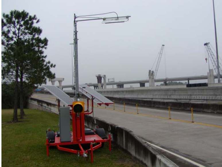
Figure 9. Relocated Mobile AVI Violation Enforcement Unit Northwest Transit Center Exit Ramp
